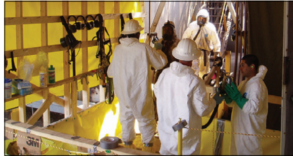
Measures that Protect Workers (L) Protective clothing and equipment (R) Dosimeters track workers' exposure. Signs and barrier tape denote areas of contamination and whether a work permit is required.
