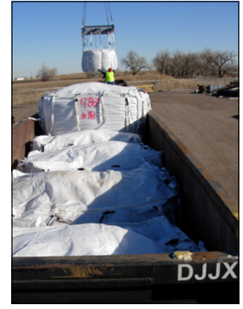
Waste Loading Loading SuperSacs in EnergySolutions' supergondola railcars
